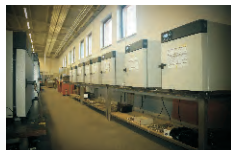
3rd production hall 1 948 m 2
